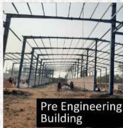
Pre Fab Structure
